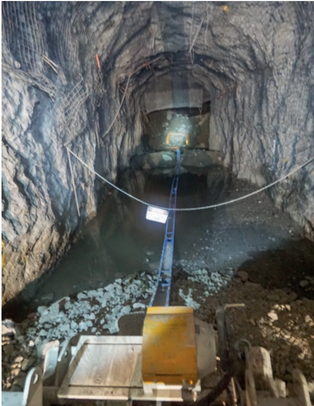
6. As the extraction commences, the pressure is applied slowly to the connecting racks and tow sling.
