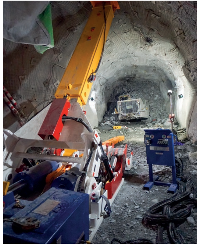
12. View of the buried asset from the rear of the MED360.
