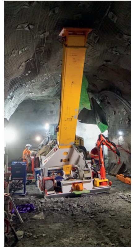
8. Boom and head plate positioned into the roof of the tunnel.
