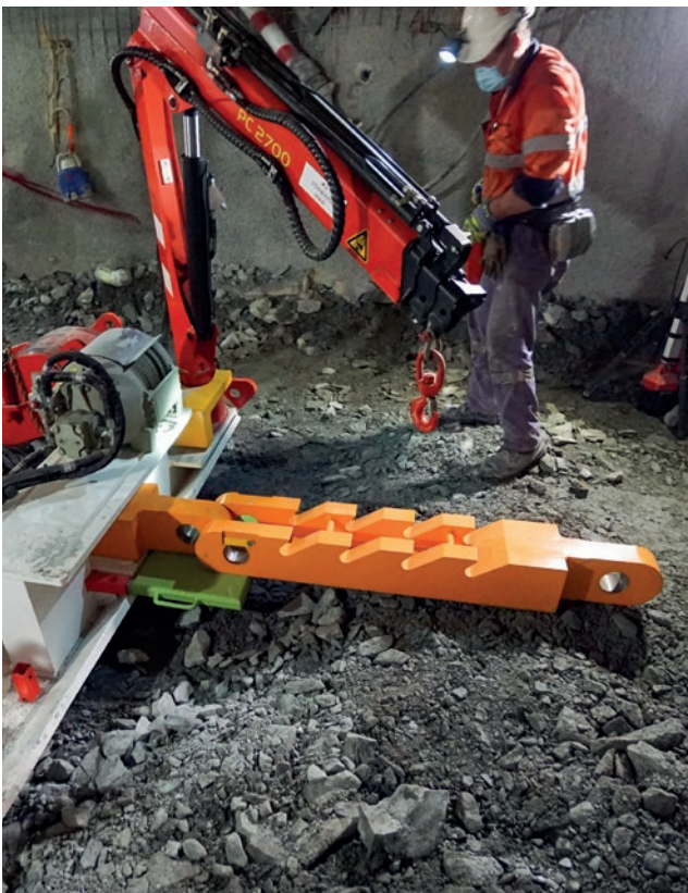
9. Racks are being located and pinned together using the front Hiab. (Hiab cranes are only available on the MED360).
