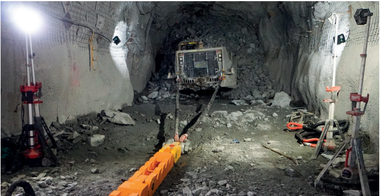
16. Tension is applied to the tow slings and the extraction process commences.
