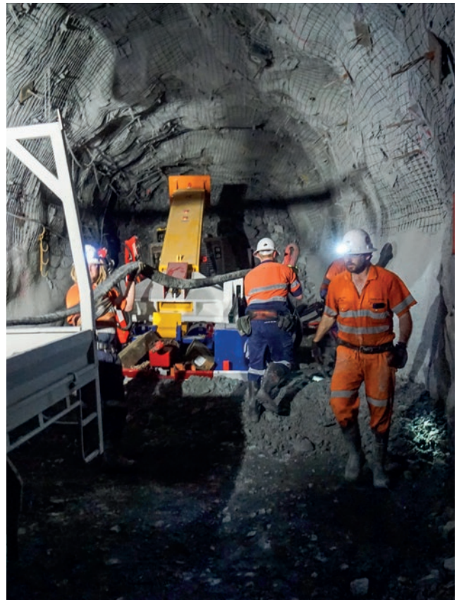
3. The tow slings and other equipment are moved into position.
