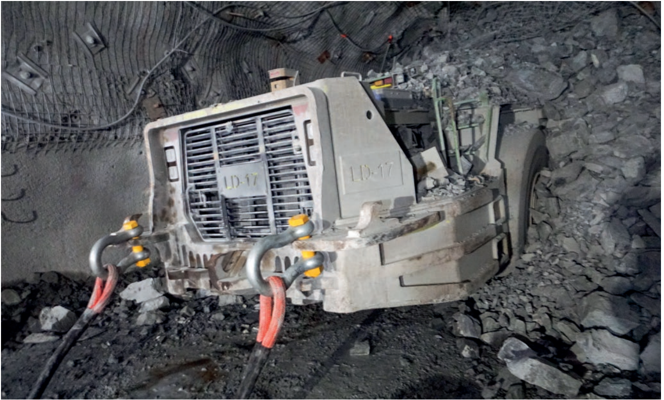
15. The tow slings are attached to the 'D-shackles' and readied for the machine extraction.
